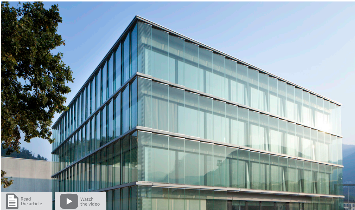
The five-storey office block has been built to meet the Minergie Eco standard and offers a total surface area of 2600 square metres (Image: CSCS)
