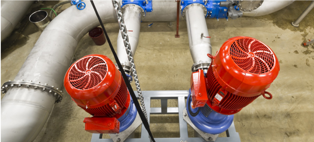
Powered by the water circuit as it flows back toward Lake Lugano, these two micro-turbines in the pumping station produce an extra 200 megawatt hours of energy per year. (Image: CSCS)
