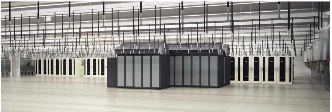
Rendering of the machine room with supercomputers in the foreground and cooling islands for additional hardware in the background.
