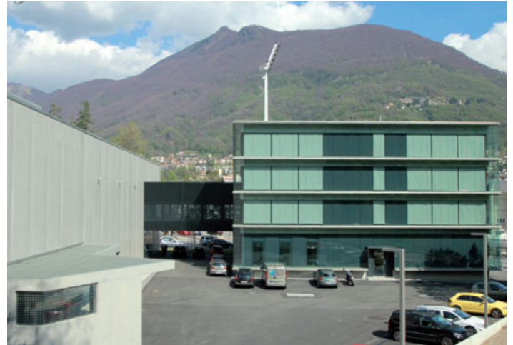
The computer building (left) and the office block (right) are connected by a bridge and an underground tunnel. (Picture: CSCS)
