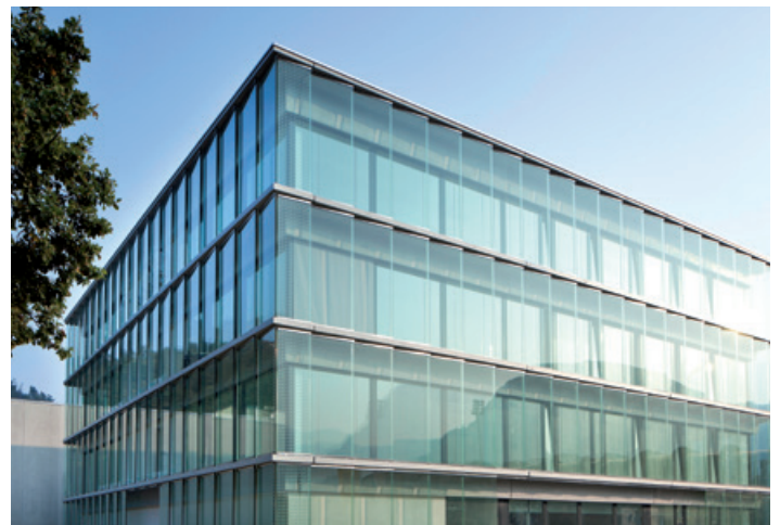
The office block with its distinctive double layered glass facade. (Picture: Marco Carocari)
