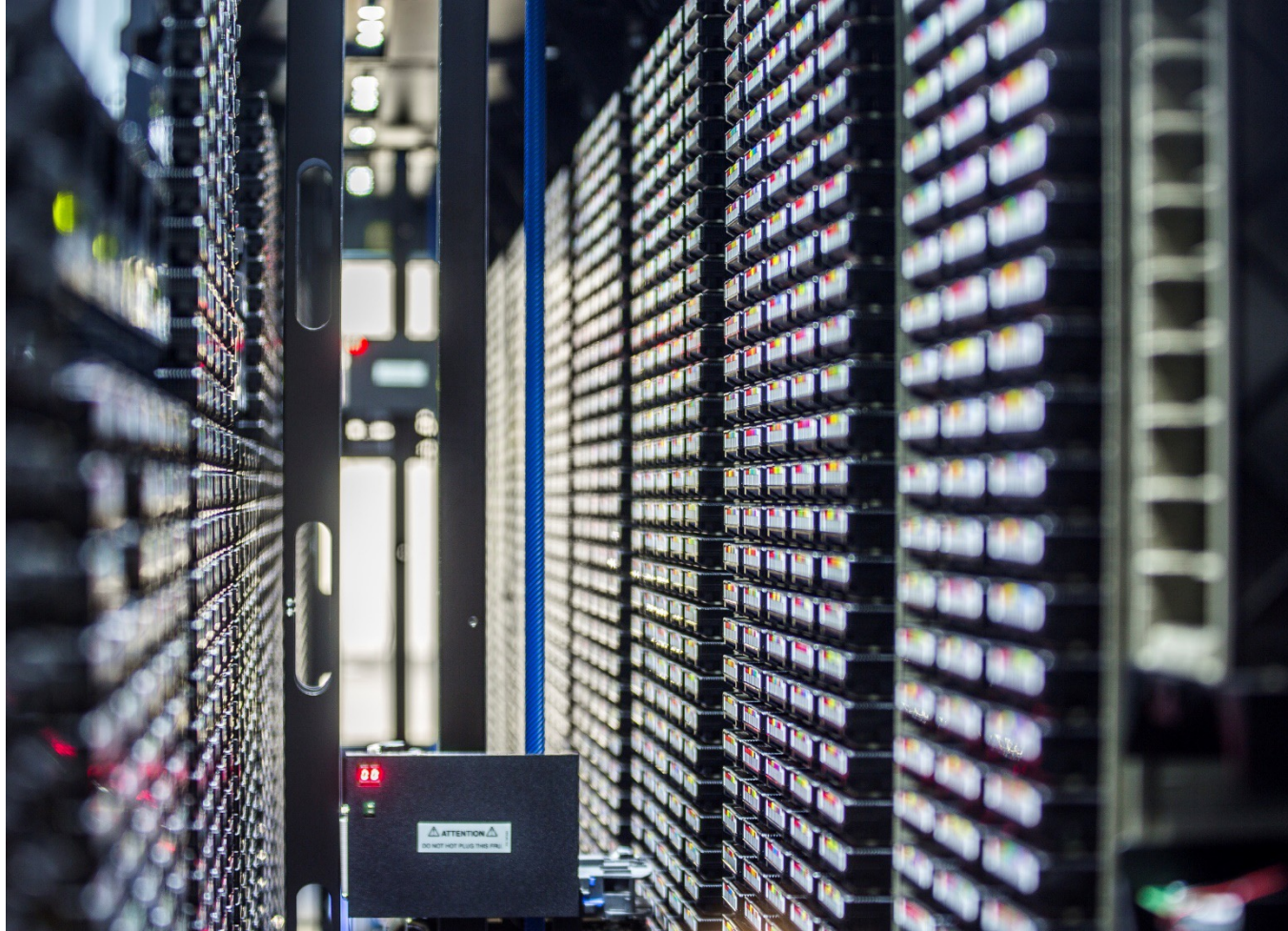
Inside the CSCS tape archive
